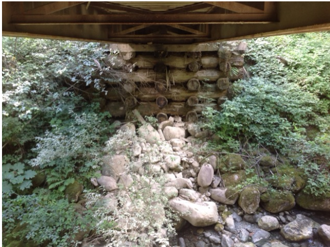
Right Bank Abutment when facing downstream
