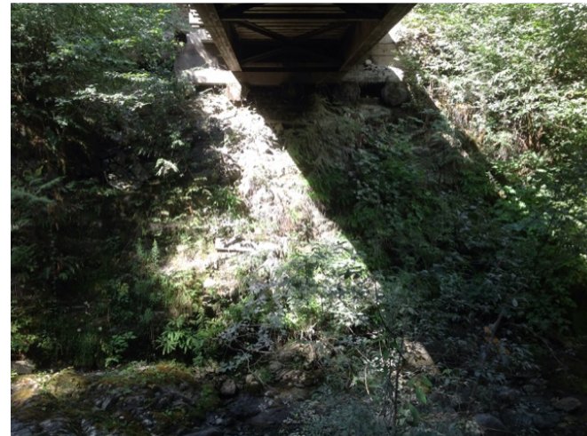
Left Bank Abutment when facing downstream
